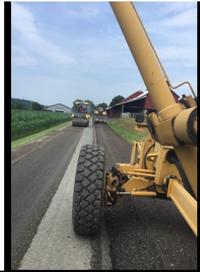
Road Reclamation/Grinding
