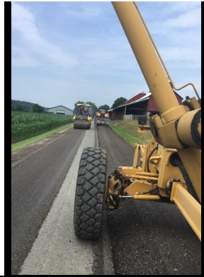
Road Reclamation/Grinding
